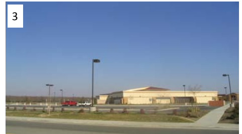
Main Building Exterior Lighting
