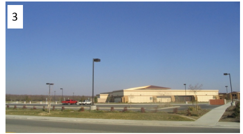
Main Building Exterior Lighting
