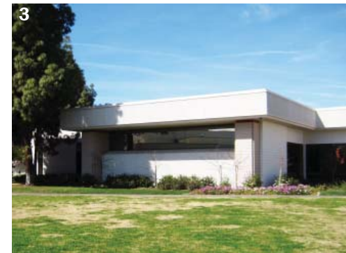
3 1980's LRC Building 4 Pedestrian Gateway
