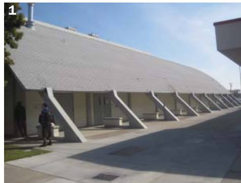
1 1960's Gymnasium 2 Health Careers Modular Buildings
