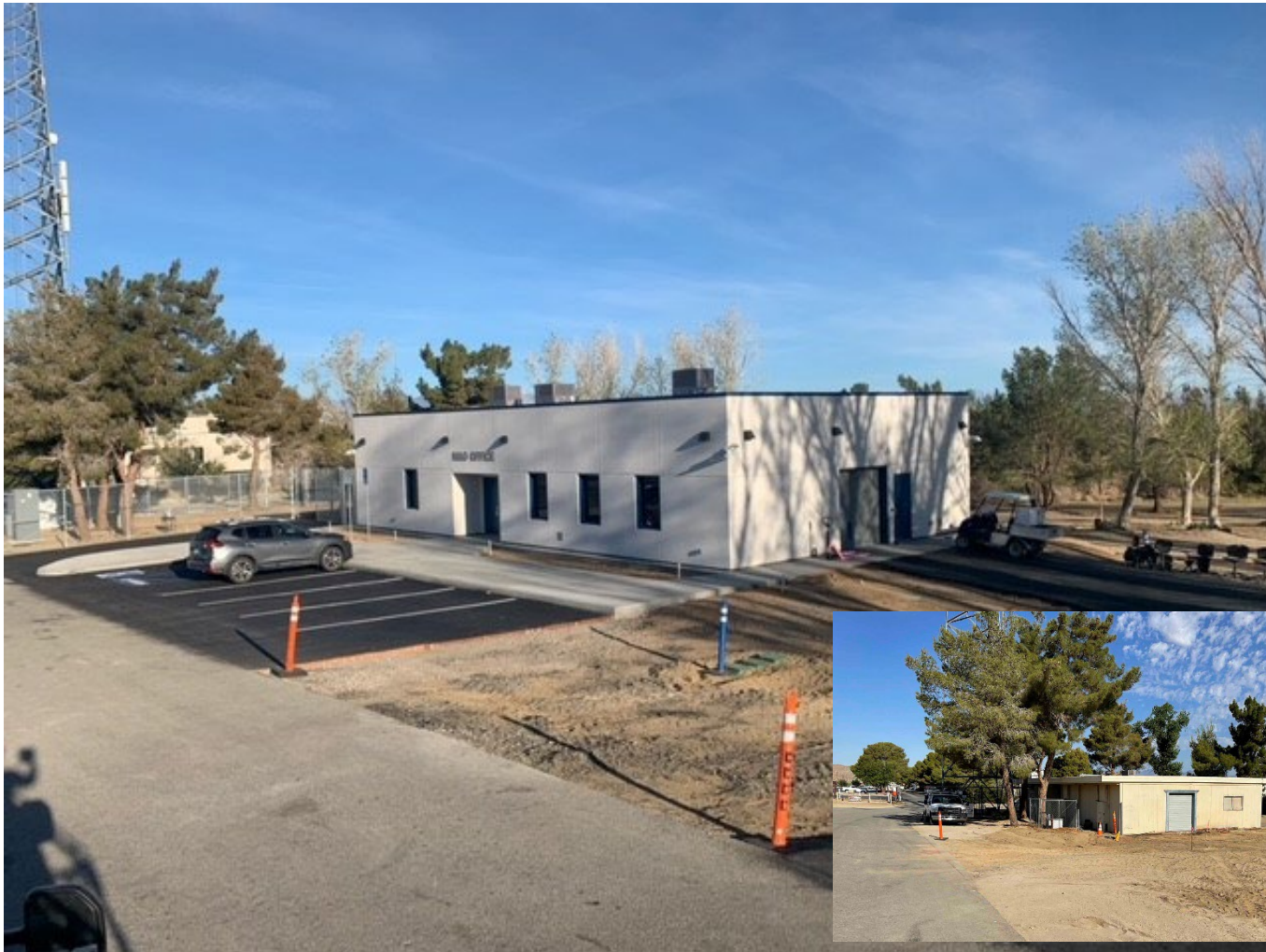
New M & O Facility - Complete – January 2022
