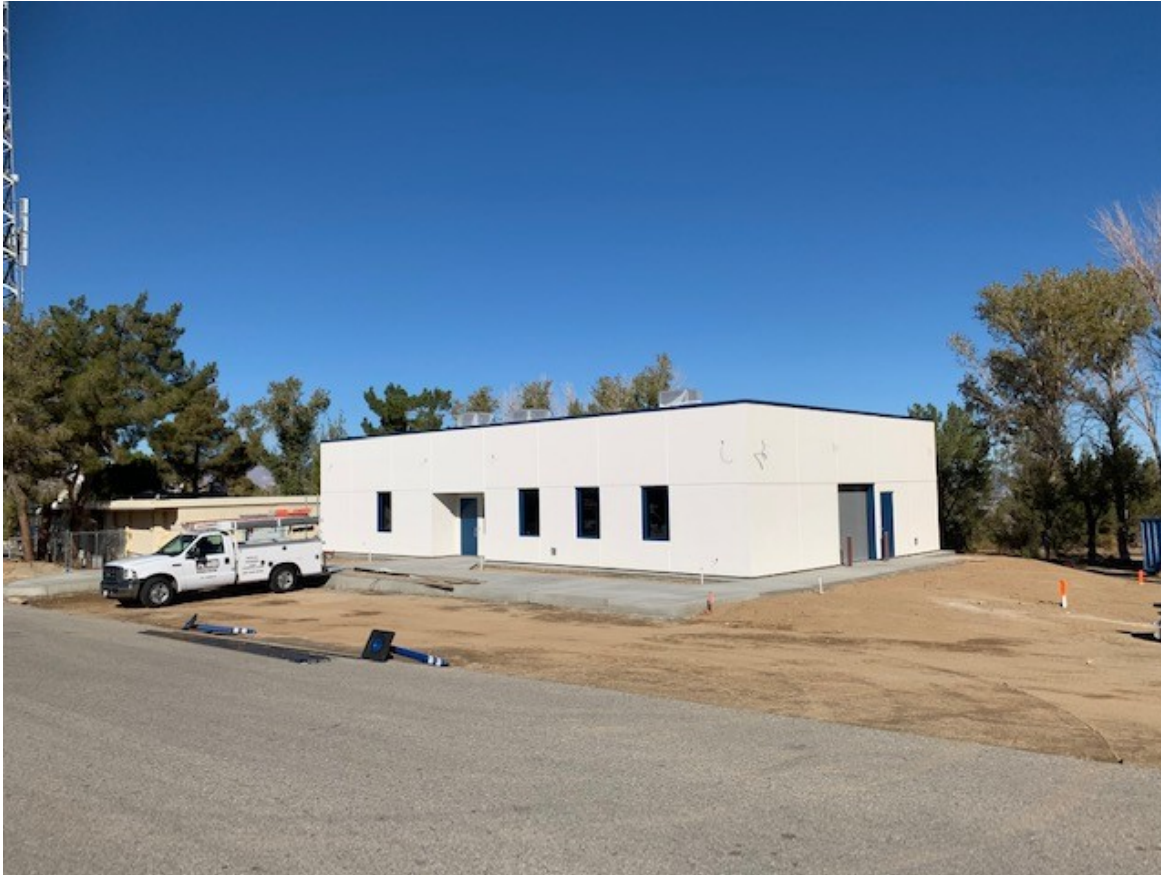
New M & O Facility - Under Construction
