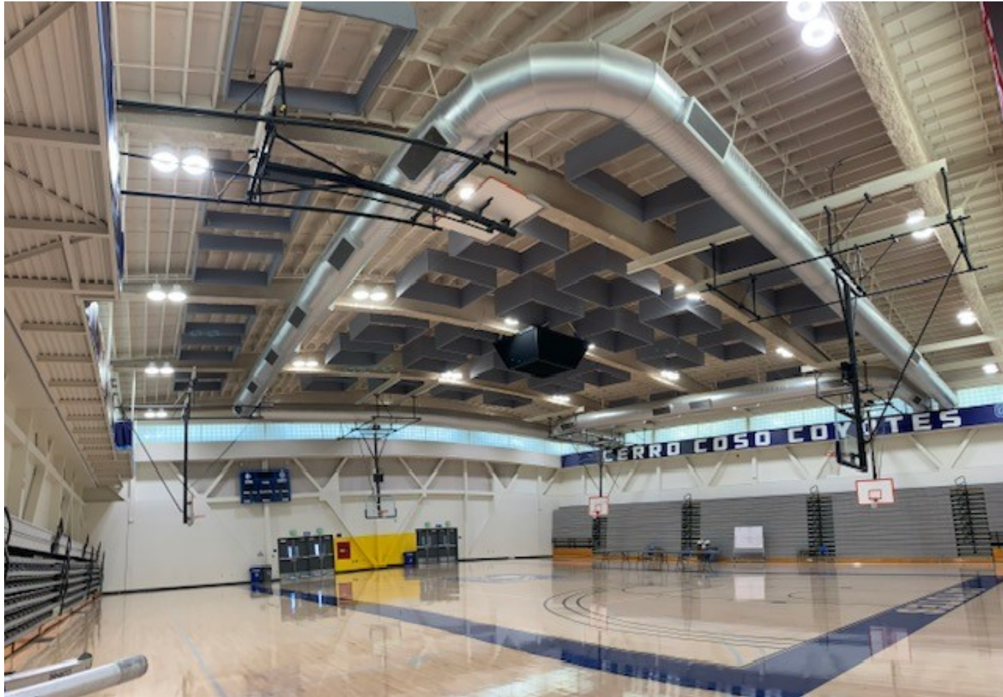
Gymnasium Lighting and Building Upgrades
