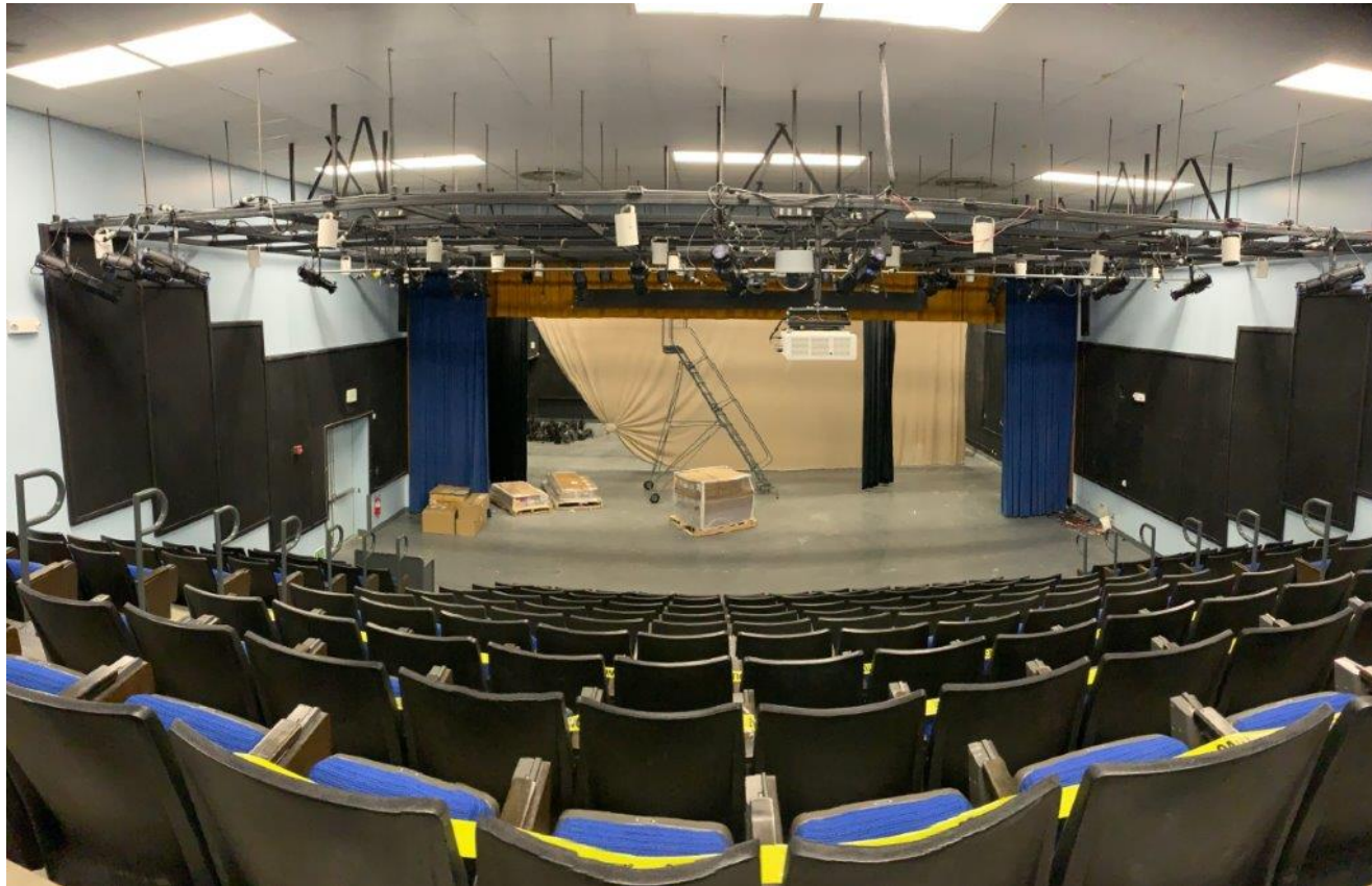
Main Building Lecture Hall Renovations
