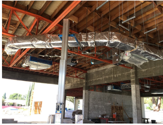
ABC Building/Campus Student Center Modernization
