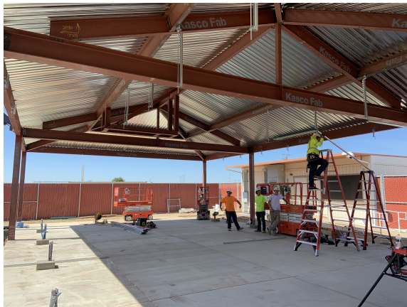
Delano HVAC Lab
