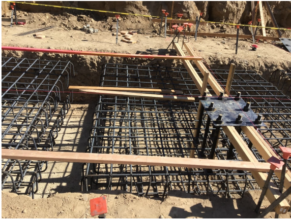
ABC Building/Campus Student Center Modernization
