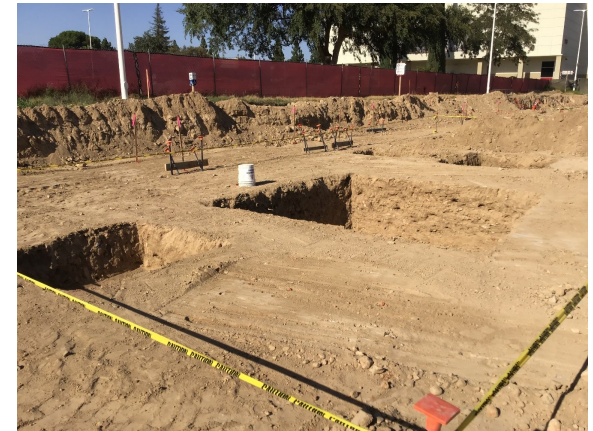
ABC Building/Campus Student Center Modernization
