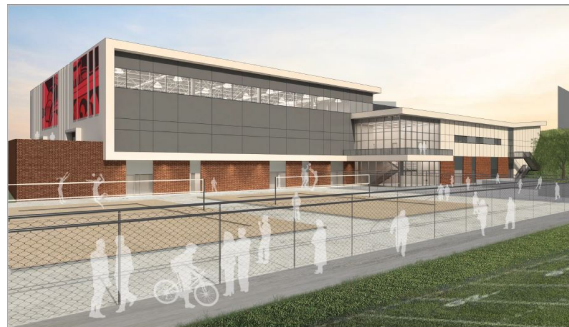
Combined Gym and Fieldhouse
