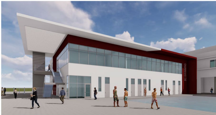
EXTERIOR VIEW - POOL BUILDING - SOUTH-WEST KCCD BAKERSFIELD COLLEGE POOL BUILDING FEASIBILITY STUDY
