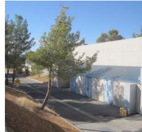
IWW- Service / Shared Pedestrian Access
